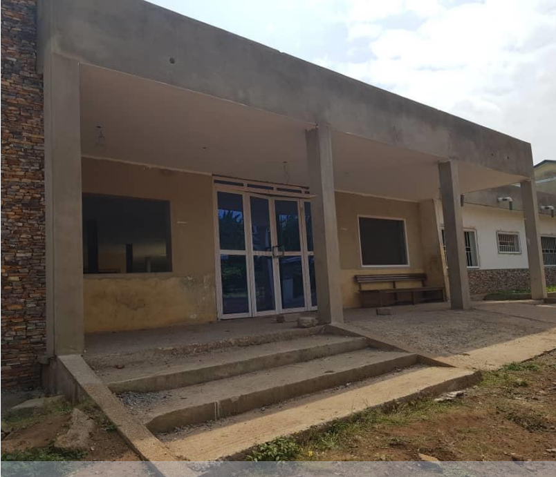
REHABILITATION OF LARTEH CLINIC
